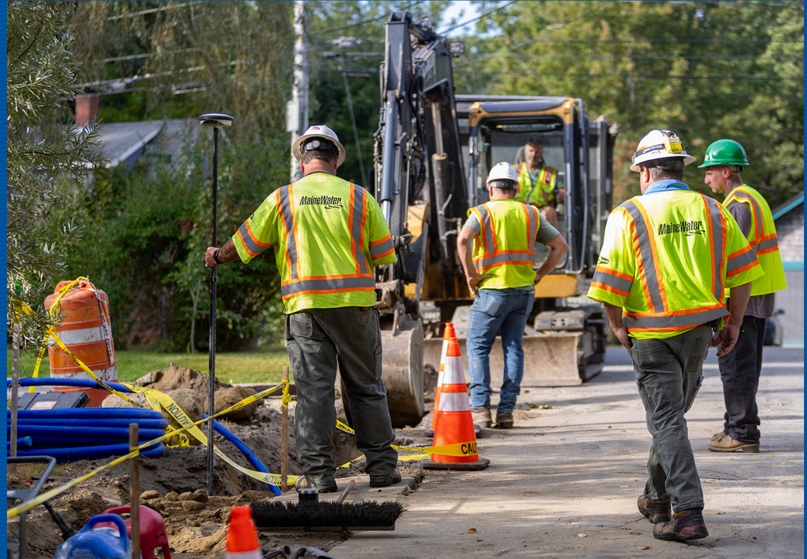
A water main replacement project in the Camden-Rockland area in Maine.
